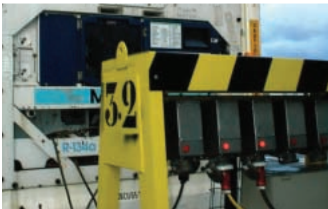
A reefer plug application at the port of Dunkirk, France
