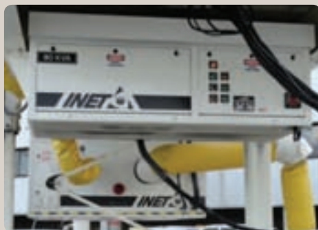
Bridge Mounted 400Hz static converter in action at an airport in USA.
